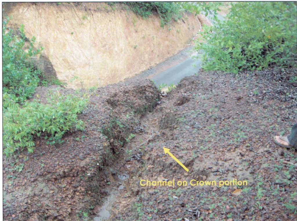
Photo 7: channels made for property demarcation on the crown portion of the slide from which water is directly draining in to the slide area.
