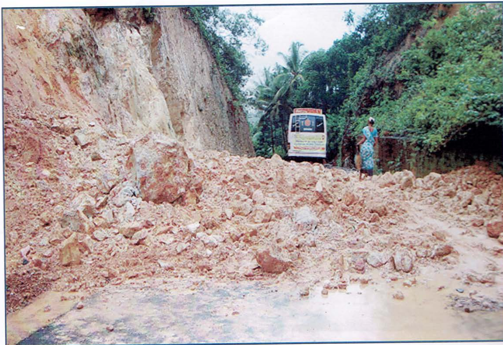
Photo 2: View of the landslide near Onibagilu on Peruvai- Pakalkunja road connecting Vittla and Manila on 21.07.2010(a day after the slide). courtesy daijiworld.com
