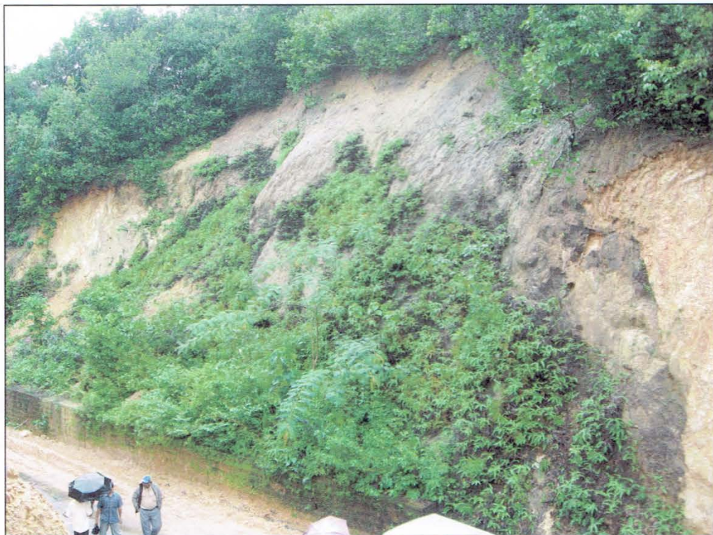
Photo 8: view of the landslide on the other side of the road which has been stabilised by providing retaining structure and slope grading.
